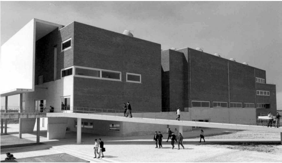
Figure 2: The eastern façade
