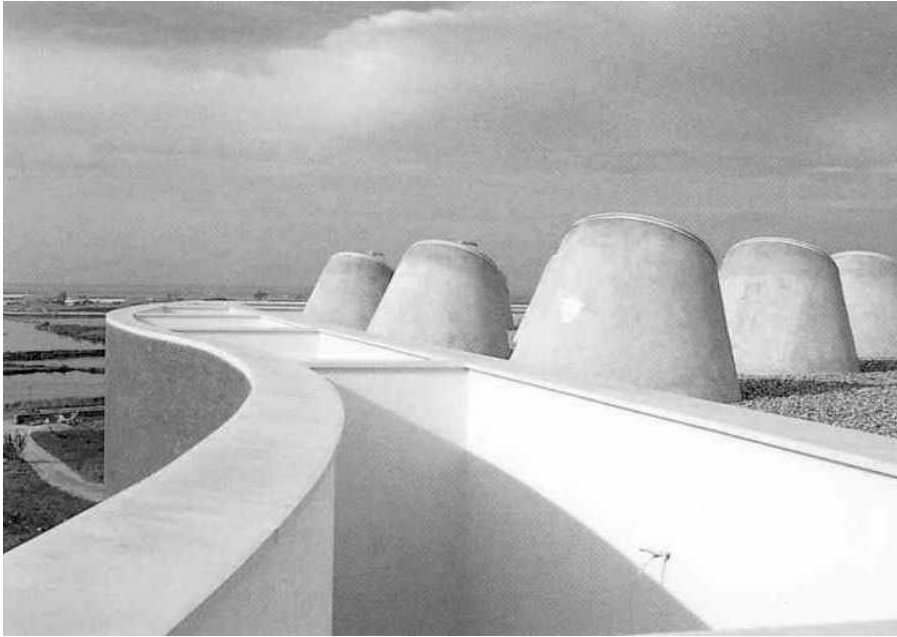
Figure 4: The roof clerestories
